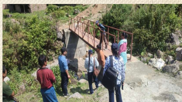
Steel foot trail culvert
