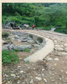
Bhandarkhola hume pipe culvert
